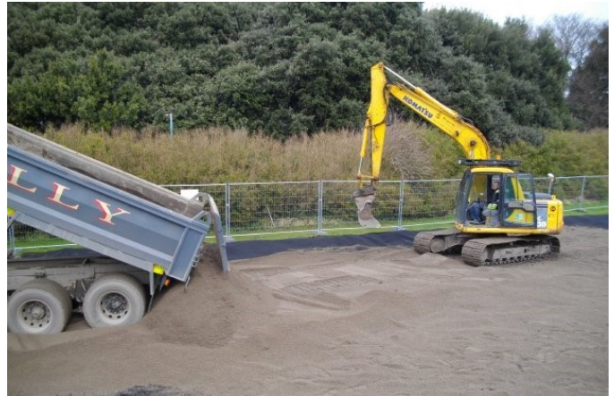
WMA—Protecting the root barrier membrane
