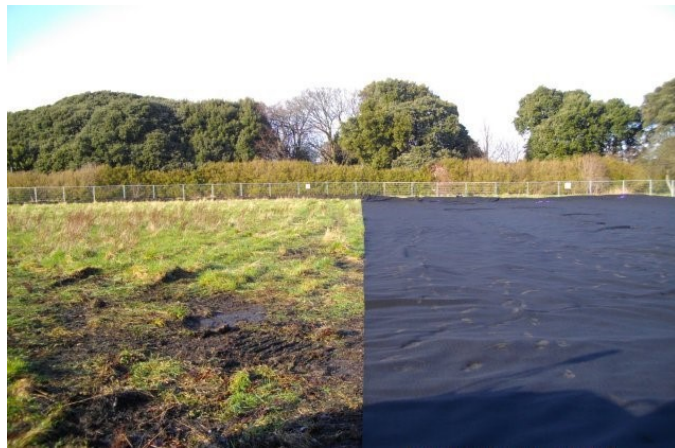
WMA—Lining before waste is stockpiled
