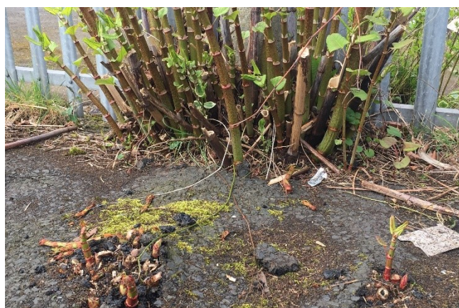
Japanese knotweed breaking through a hard surface
