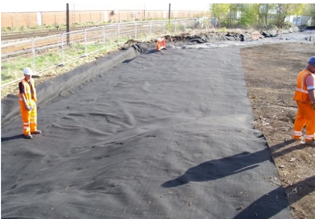
Root barrier capping
