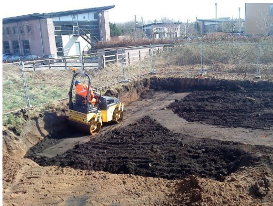
Compaction of a burial chamber
